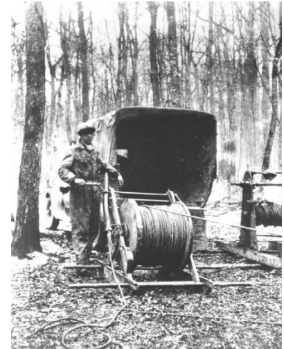
First electrical well log, Pechelbronn, France, September 5, 1927
