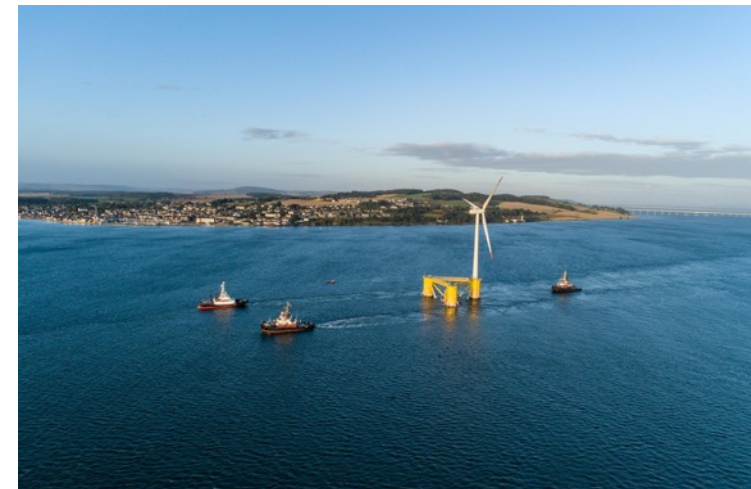
Tug supply vessels towing Kincardine floating wind turbine →
