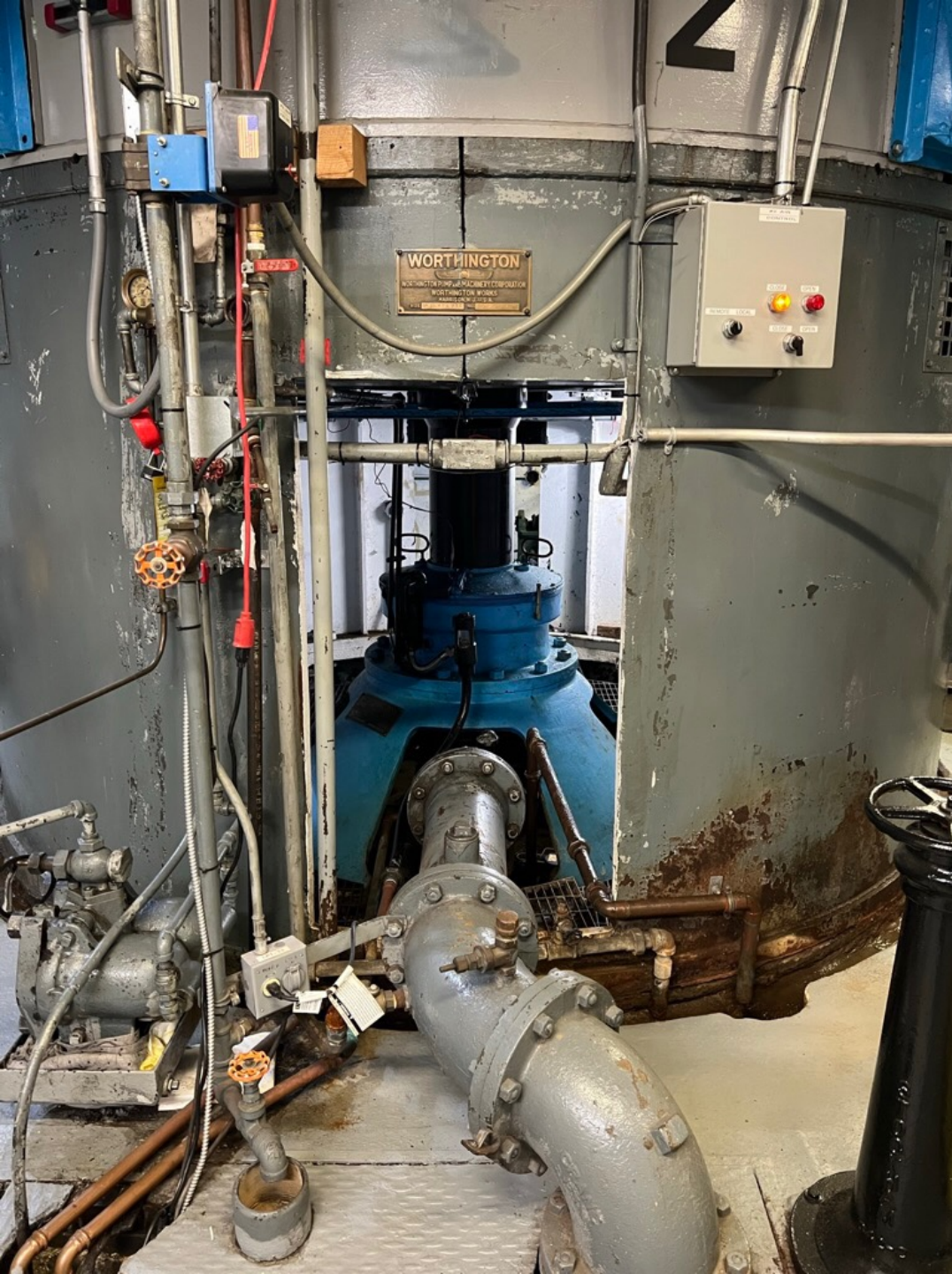
← 1 of 2 pumps, which also run as generators adding another 5MW of power capacity
